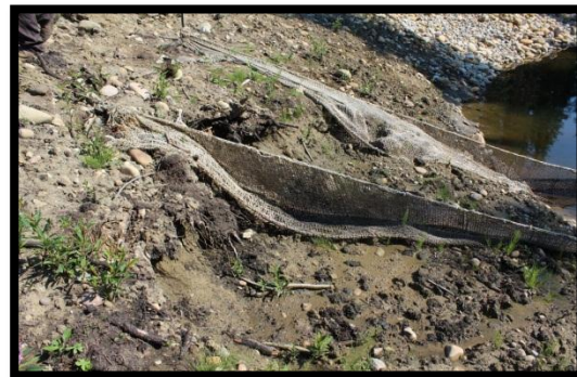
Small slump in the side slope of ST2A
