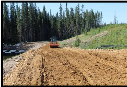
Access road grade construction at ST2A
