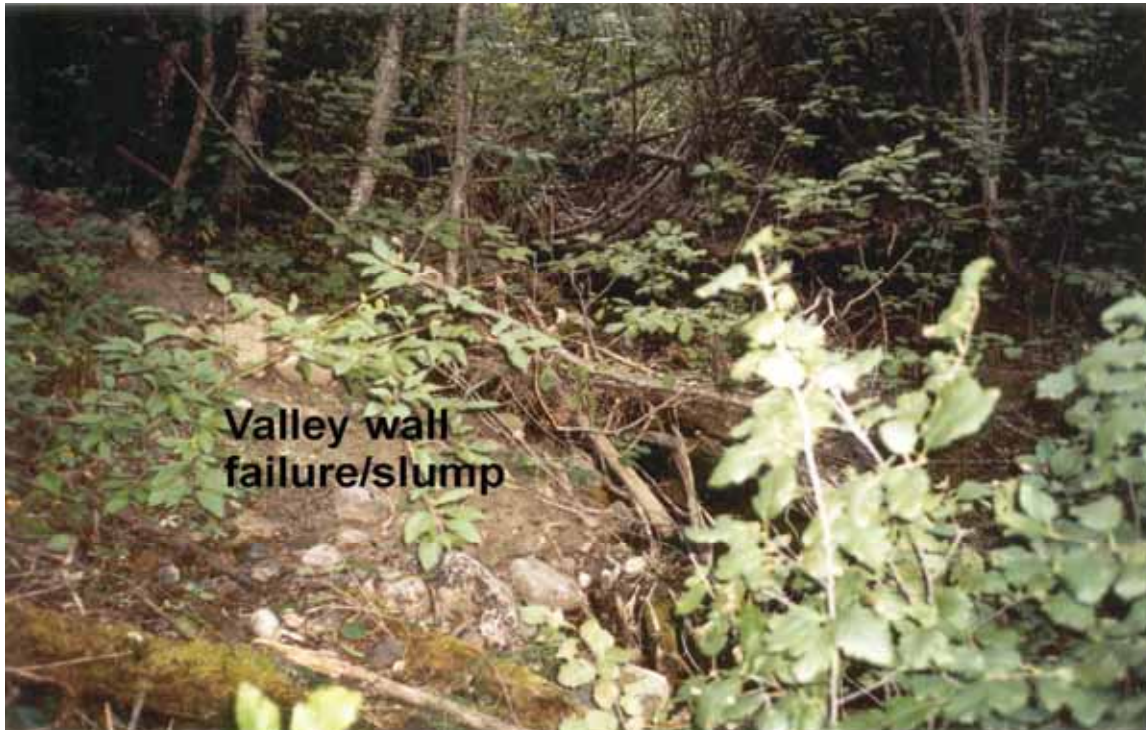
Plate 1. Valley wall failure/slump into Canyon Creek tributary upstream of population estimate section.
