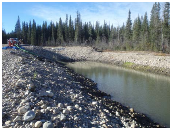
Plate 6. Looking upstream across the downstream cell of Sediment Trap 3.
