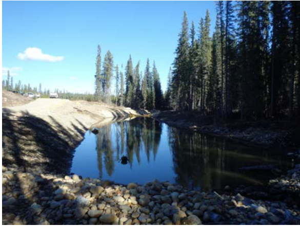
Plate 1. Looking downstream at Sediment Trap 2A after the jute curtain removal.
