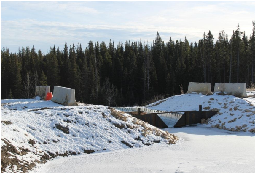
Completed ECP Weir and Culvert Repair: Installation of ½ Round Culvert
