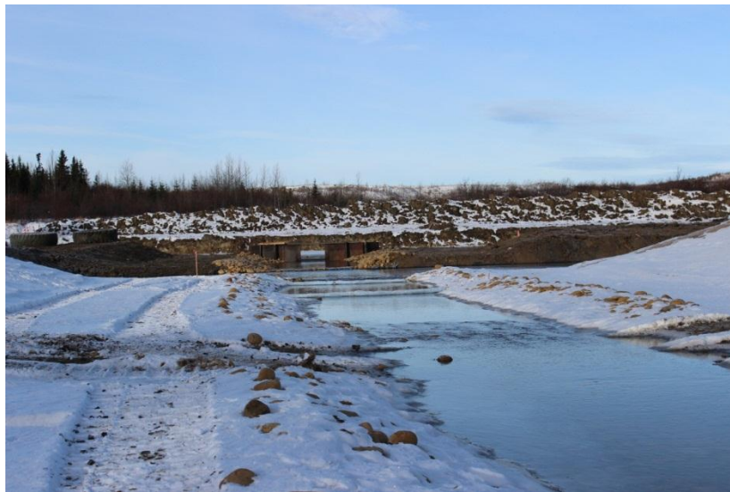
Main Tailings Pond Spillway with flow, Rectangular Weir in Background
