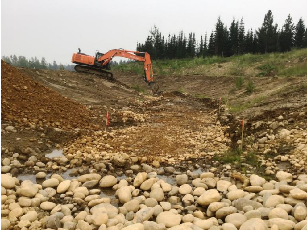
August 14, 2018: Looking downstream at channel shaping from 0+250 to 0+290 and pitrun gravel placement on channel bed from about 0+240 to 0+270.
