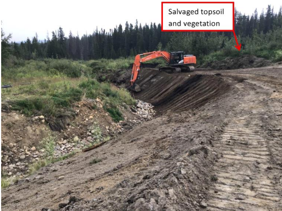
August 17, 2018: Looking downstream from 0+360 at shaping of right overbank.
